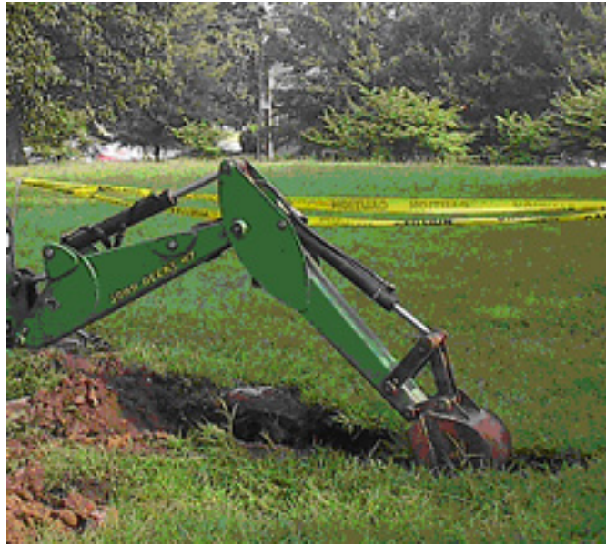
Figure 1: Trenching with the John Deere Model 47 Backhoe
